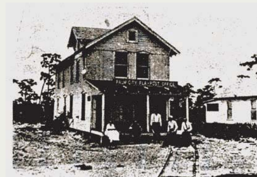
Original Palm City General Store and Post Office
