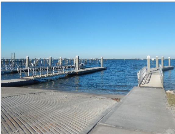
Image 14 The exemplar accessible courtesy dock at Jensen Boat Launch Ramp.
