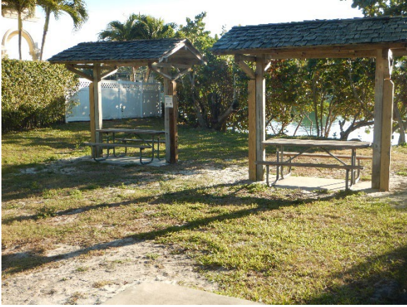
Image 12 The picnic pavilions at Porter Park lack an accessible route and tables with wheelchair accessible seating.
