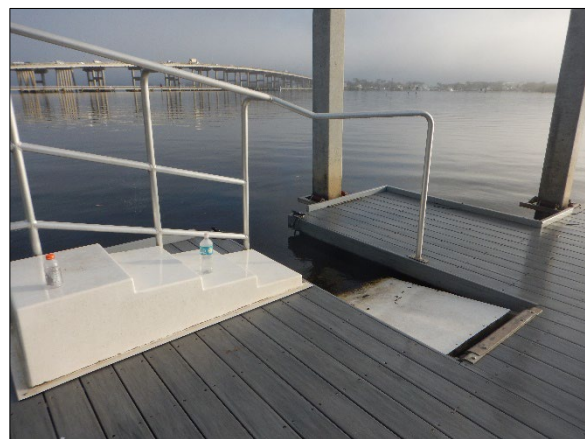
Image 17 The AccuDock Safe Launch and transfer platform at the Rowing Club at Charlie Leighton Park.
