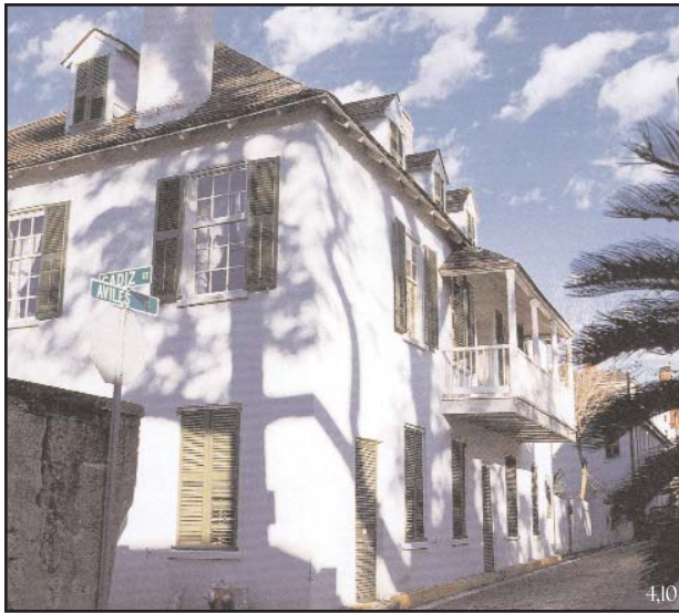
XIMENEZ FATIO HOUSE, ST. AUGUSTINE, FL: This early St. Augustine house reveals the truly urban character of the old city. The house is brought directly to the street, and a projecting balcony encroaches onto the roadway/sidewalk. This type could be adapted to accommodate a mixed-use program.
