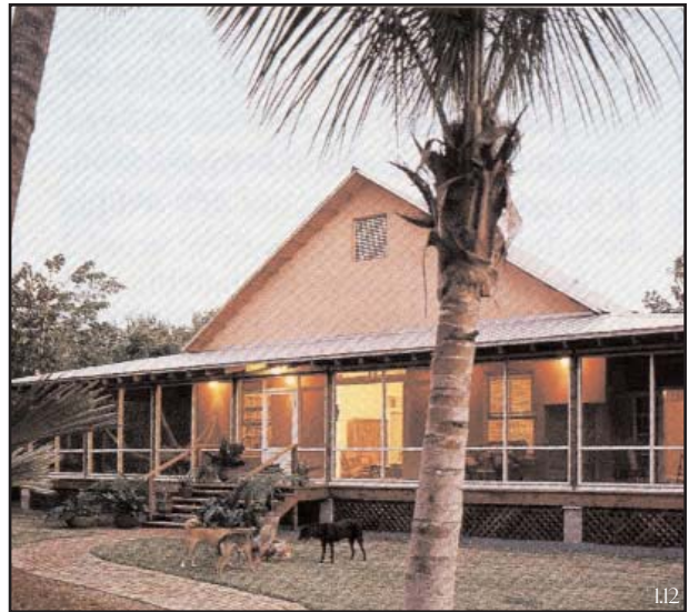
FLORIDIA, MIAMI, FL: Florida is a contemporary version of the cracker style by dLGV architects. The predominant features of the house are the large screened wrap-around porch and the steep pitched gable roof. The entire house is raised above grade to vent the substructure and to allow flooding to occur during storm showers and surges.
