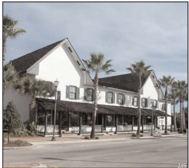
MIXED USE BUILDING: Florida wood-framed vernacular is not limited to single-family homes. In this Florida example, a mixed-use building is influenced by the style. The composition combines two gable-ended structures connected by a lower mass and tied together with a continuous porch.
