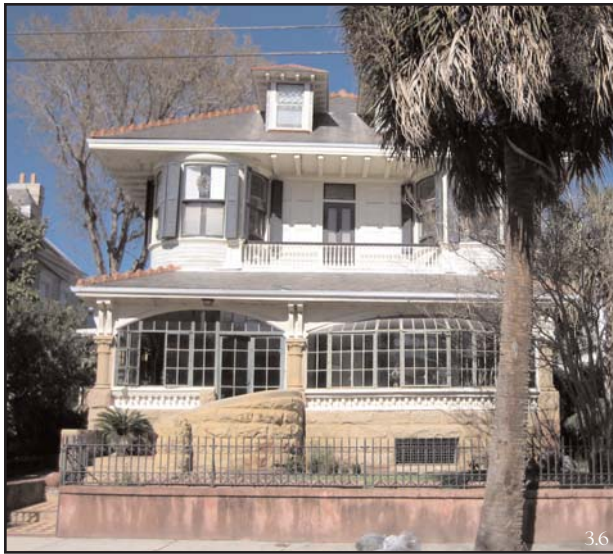
HOUSE, CHARLESTON, SC: Pictured above is a somewhat eclectic version of a Carolina bungalow. The porch has been filled in, but the its impression is still felt. An upper story porch is added to connect two projecting bedrooms. A large overhang with a simple plank soffit cover the house. The dormer above reveals an attic story.
