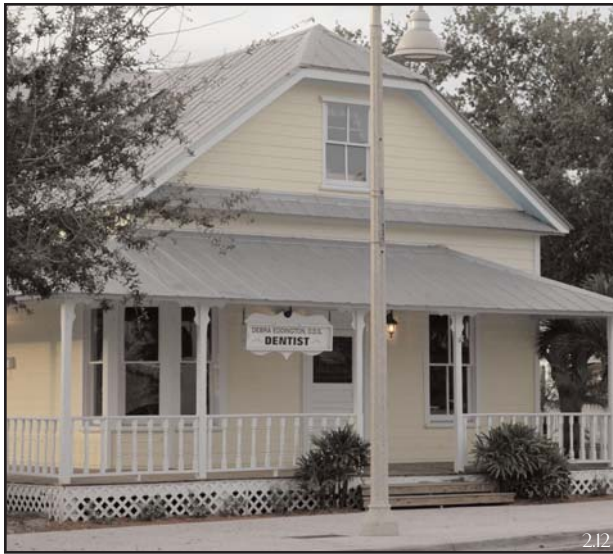
DENTIST OFFICE, JENSEN BEACH, FL: This beautiful example of the wood-framed vernacular is located in downtown Jensen Beach. Originally a single family home, it building has been converted to accommodate a dentist office. The textured siding and hipped gable ridge are variations to the style.
