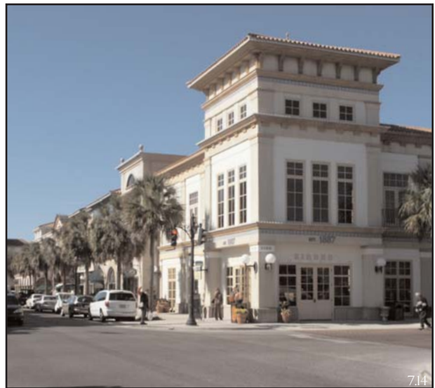
COMMERCIAL CORNER, VILLAGES, FL: This mixed-use building in the Villages, Florida emphasizes the strength that additional height at the block corners can have. In this case, the additional height of this classically inspired Mediterranean building is articulated in the building itself with a corner tower element.
