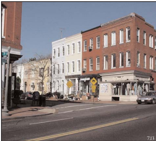
COMMERCIAL CORNER, GEORGETOWN, WASHINGTON, DC: In mixed-use districts that encompass several blocks, the corners should be encouraged to be built to slightly greater heights. The added height helps to contain the wider width of the intersection and creates awareness of the commercial activity held within.
