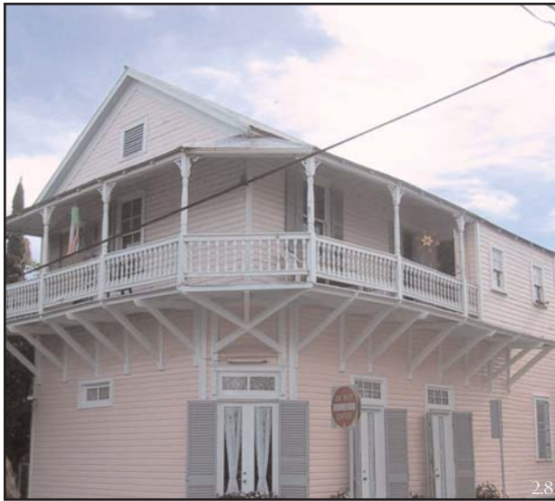
CORNER HOUSE, KEY WEST, FL: This Florida vernacular Key West home emphasizes the corner by chamfering the lower floor to face the street and wraps the porch around the two urban sides on the upper floor. Although most examples are symmetrical, it is not a rule, and this example shows a clever contextual response.
