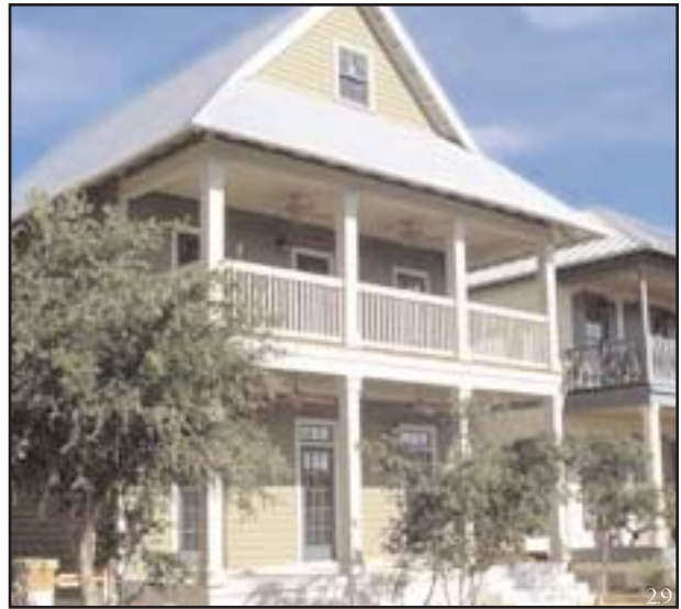
HOUSE, ROSEMARY BEACH, FL: Above is a very typical Florida wood vernacular home. Stacked porches are the main ordering element in the facade. A gable roof is oriented perpendicular to the street. This is typical of the style, although the gable can run parallel as well. The attic is occupied with an additional bedroom.
