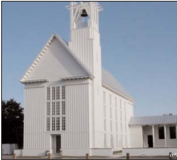
CHAPEL, SEASIDE, FL: The chapel in Seaside maintains the wood framed vernacular of the town while differentiating itself from non civic buildings through the use of more monumental proportions, a splendid bell tower and a bright white painted finish. A provision in the town code only allows civic buildings to be painted white.
