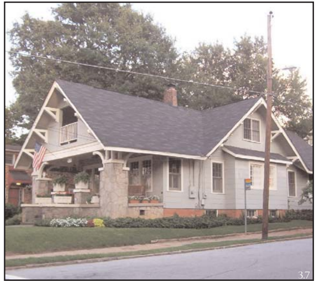
HOUSE, ASHVILLE, NC: Roof brackets are a common feature of the bungalow style. Functionally, they are needed to help support the massive room overhangs' aesthetically, they are often elaborated and become beautiful objects that help give a strong character to the house, as is the case in this North Carolina home.
