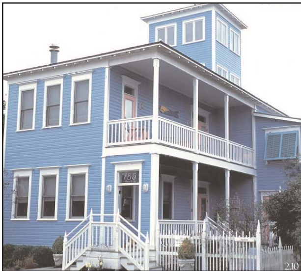
HOUSE, SEASIDE, FL: Seaside contains countless contemporary Florida vernacular homes, all with different interpretations of the style. Here, a side yard typology is utilized with a tower bedroom added to the composition. White corner boards provide contrast to the rich blue paint scheme. The entrance is clearly articulated.
