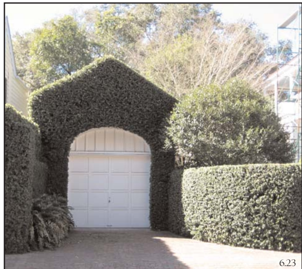
GARAGE, CHARLESTON, SC: This garage is set back from the street and heavily camouflaged by neighboring vegetation and a manicured ivy covering. Again, it is not a desirable condition to present a garage to the street, however, if it is unavoidable, then a solution such as this, is acceptable.
