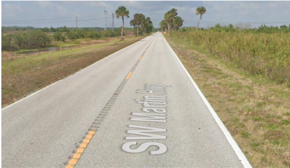
Example of Rumble Strips on SW Martin Highway
