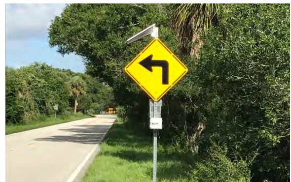
Example of Low-Cost Treatment for Horizontal Curve Safety (Source: MCB OCC)
