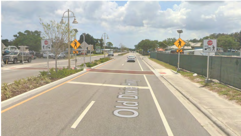
Existing Mid-Block Pedestrian Crossing on SE Dixie Highway
