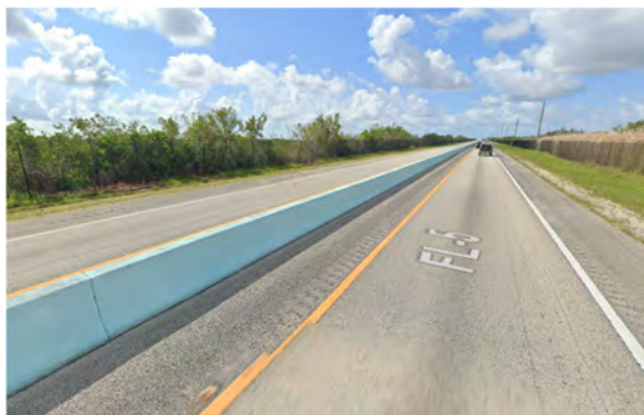
Example of Median Barrier (US-1 Miami-Dade County)
