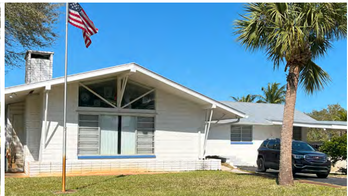
Gable roof with beams and pole brackets, Rio, FL
