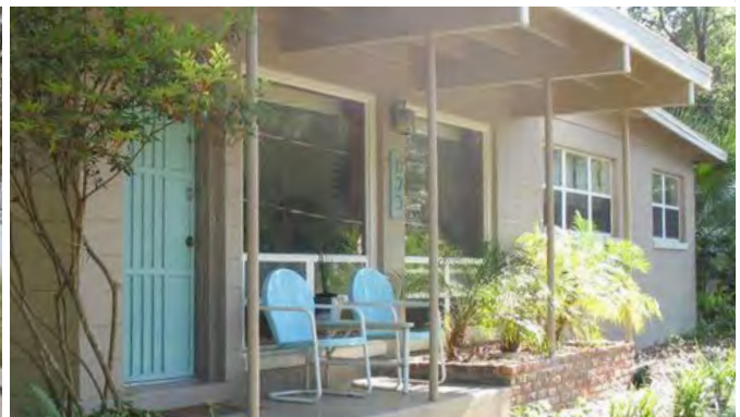
Pipe columns on a porch, Gainesville, FL
