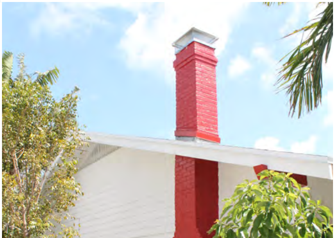
Brick chimney, West Palm Beach, FL
