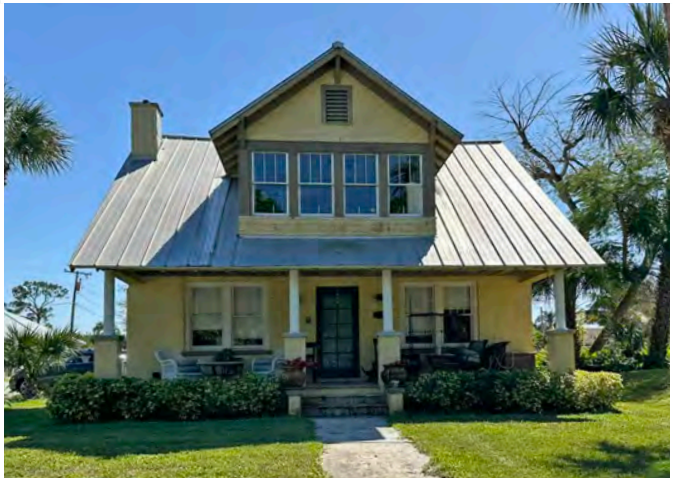
Larger dormer with shingle siding and 3 over 1 double-hung windows, Old Palm City, FL
