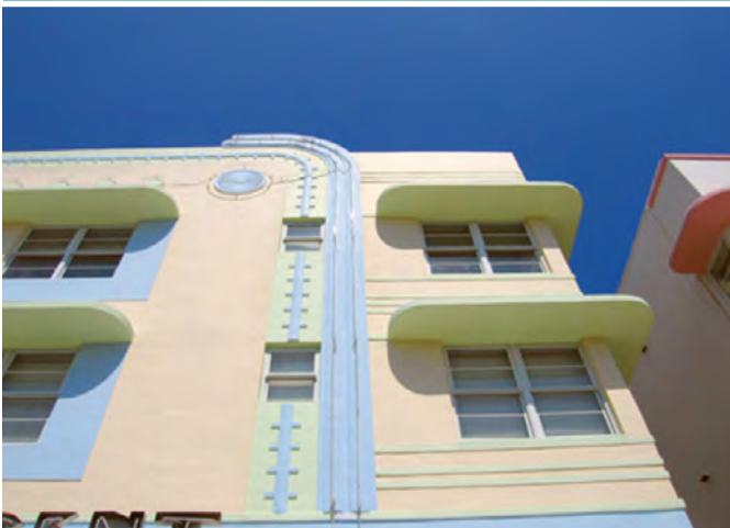
Vertical decorative facade treatment with rounded eyebrow at windows, Miami Beach, FL
