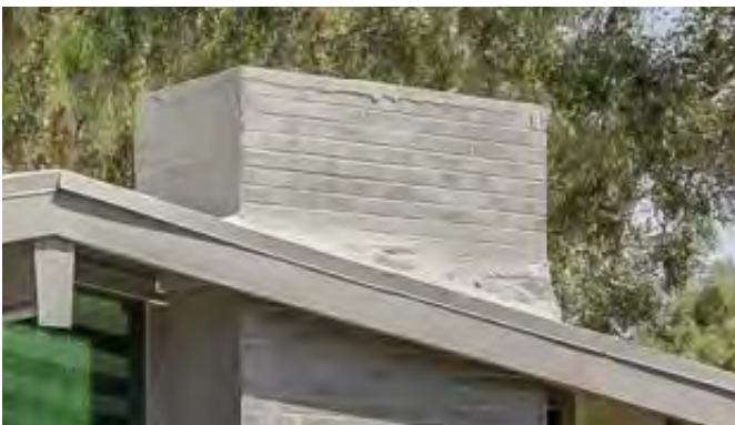
Rectangular chimney with brick facing, intersected by a gabled roof end facing the street, South FL
