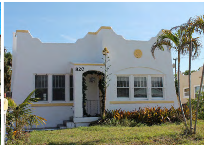
Articulated parapet on a flat roof on house in Lake Worth Beach, FL
