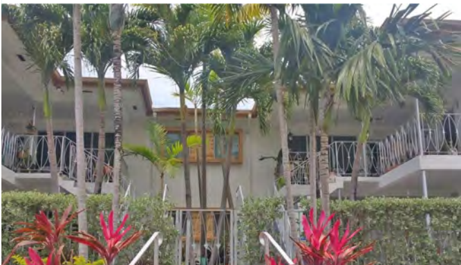
Apartment courtyard with geometric railing, Miami, FL
