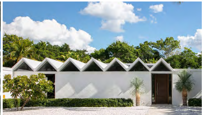
1959 dwelling designed by Ralph Twitchell, renovation by Seibert Architects, Sarasota, FL
