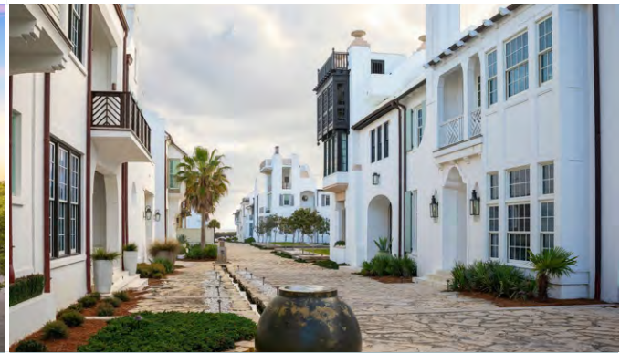
Exposed rafter tails with thin eaves, bracketed balconies; DPZ designed Windsor - Robert Orr & Associates
