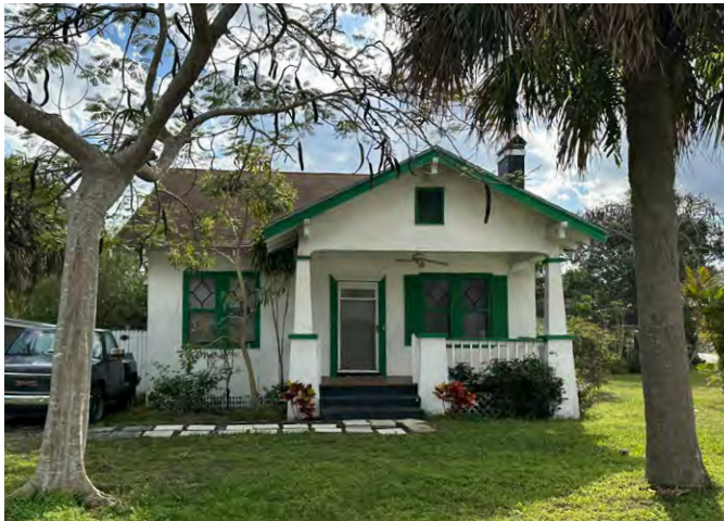
Bungalow with front porch and tapered columns, Rio, FL
