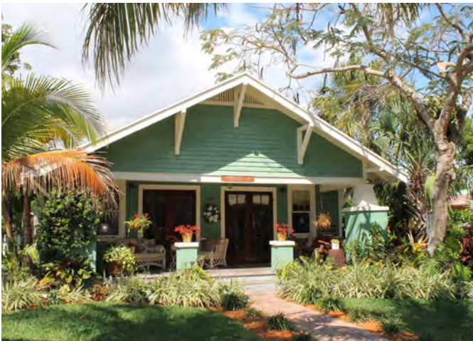
Porch with brackets, tapered columns, West Palm Beach, FL
