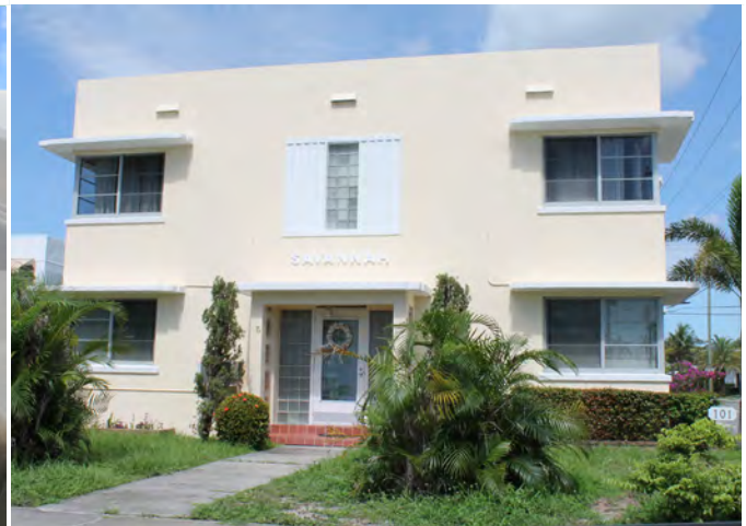
Apartment building with corner windows and deep eyebrow overhangs, South Florida
