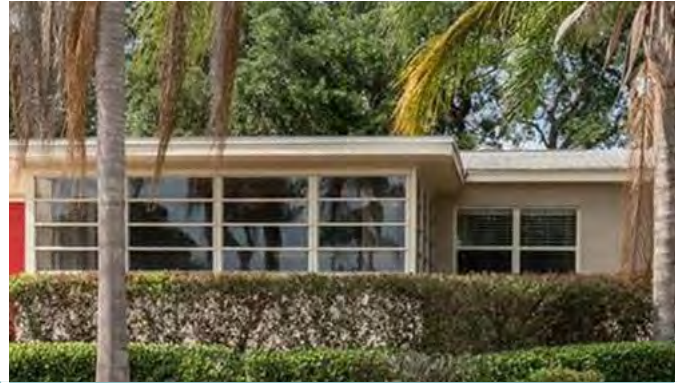
Large horizontal awning windows, Orlando, FL
