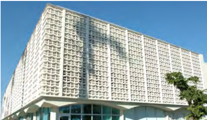
Brise soleil protects opening from direct sunlight, Miami, FL
