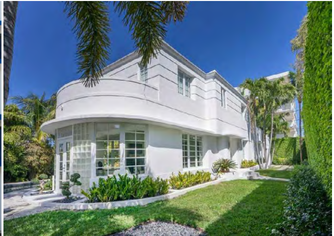
Rounded entryway ornamented with glass block and large windows with horizontal lights, Miami beach, FL
