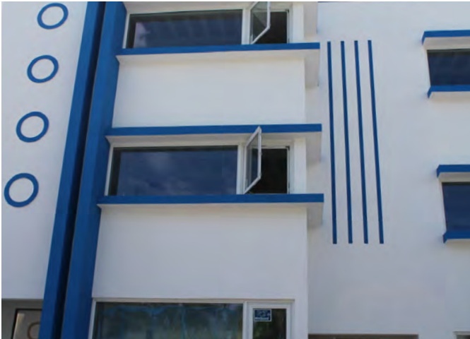
Fixed glass casement window, West Palm Beach, FL
