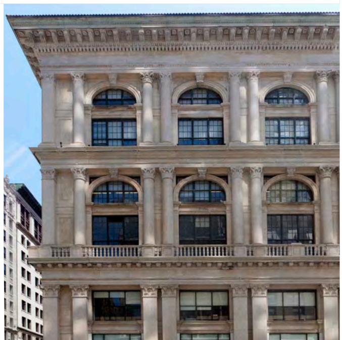
The facade is divided by large entablatures and cornices into three horizontal tiers. Tiffany and Company Building, New York, NY
