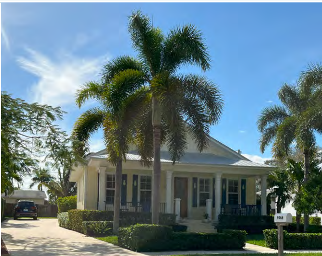
Newly constructed home with front porch, Hobe Sound, FL
