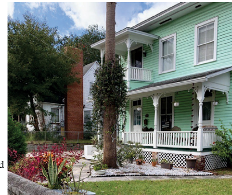
Piers with latticework. Image by ML+H.
