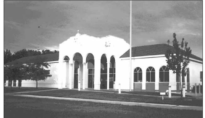
Capitals rescued from the old train station are featured prominently on the new library's front columns.
